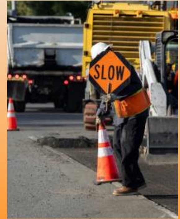
Internal Jobsite Traffic Control
