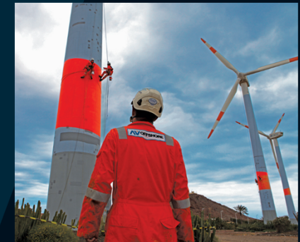
Construction Workers & Painters
